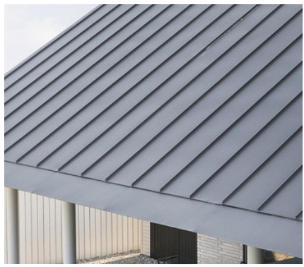
Standing seam metal roofing profile
