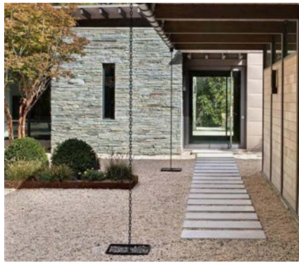
Rain chains dispatching into gravel channel
